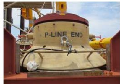
Fluid Retention Plugs Installed
